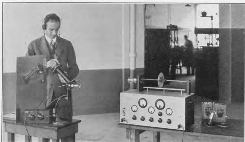
FIGURE 1. An experimental "Barkhausen" transmitter (right) and receiver (left). Mr. Karplus is measuring the wavelength of the receiver with his small reaction-type wavemeter. Two socket adapters are on the table at the right
